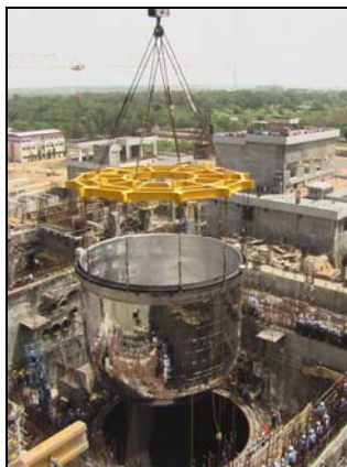
Fig. 3: PFBR safety vessel being lowered into the reactor vault
