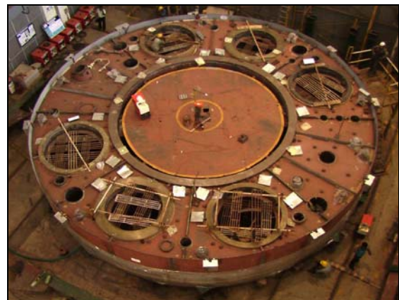
Fig. 4: Roof slab of PFBR
